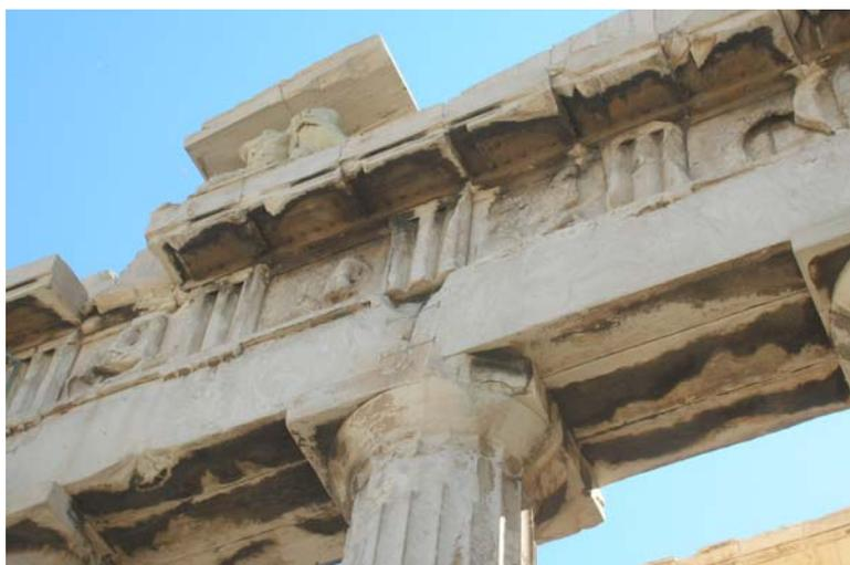
**Fig. 2.** A typical case of epistyles of the Parthenon temple connected with “I” connectors.
